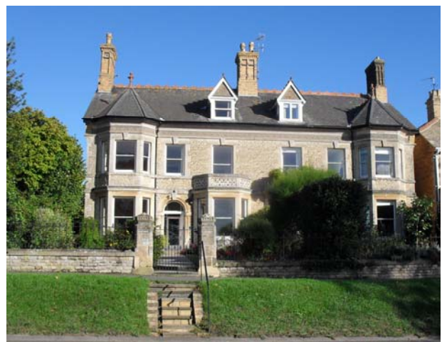
Fig. 31. Example of late Victorian houses on Tinwell Road.
