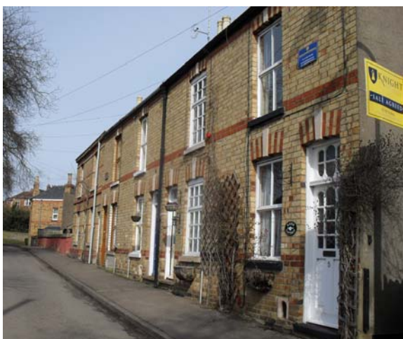
Fig. 32. Terraced housing on Water Furlong.
