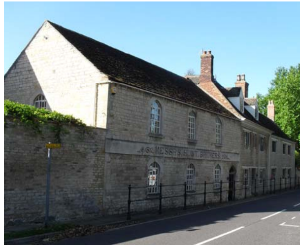
Fig. 29. Former brewery buildings on Water Street.
