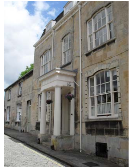
Fig. 15. Classical façade, No. 9 Barn Hill.
